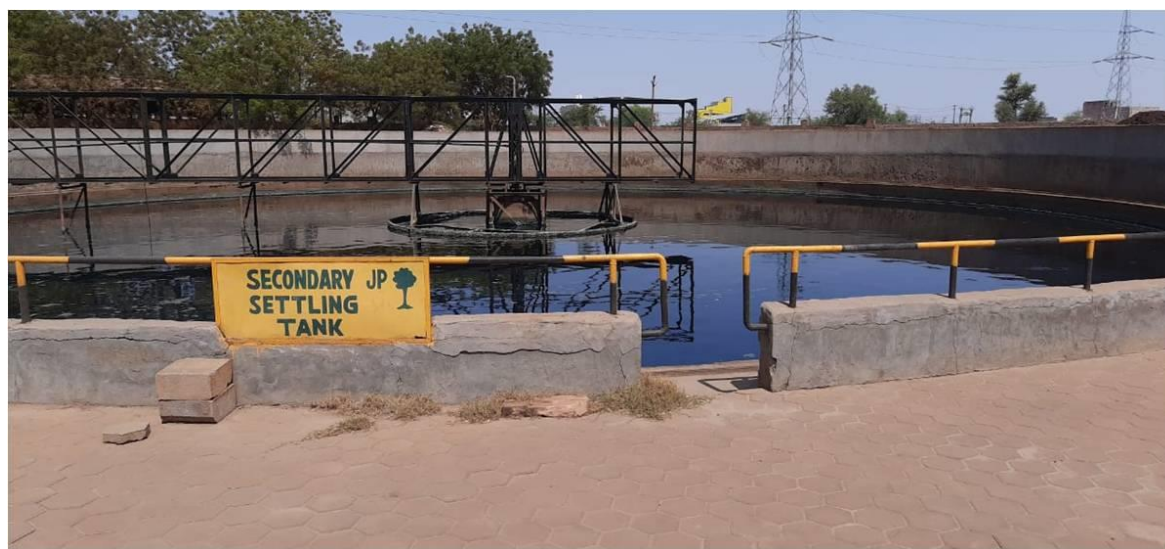
Secondary Settling Tank
